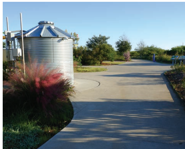
Oso Wetlands Preserve Rainwater Cistern
